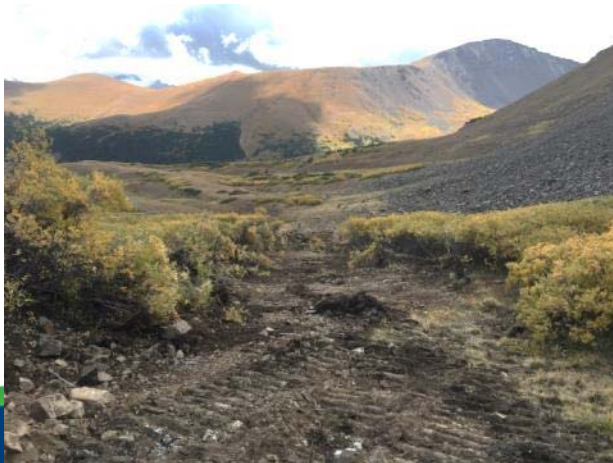
Construction of 600ft run-on-off channel
