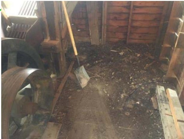
Clean-up and decontamination of Mill building interior
